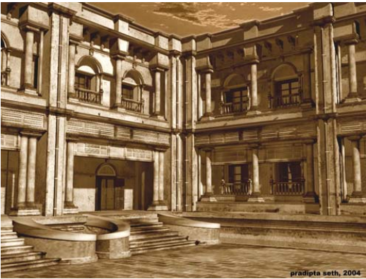
Old Courtyard Pradipta Seth
